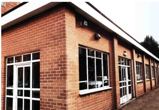
Figure 1. South Dining Hall
