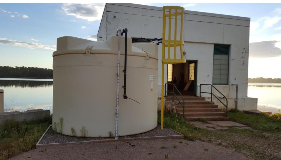
Bulk storage tank for EarthTec QZ next to intake -- 5,500 gallons
