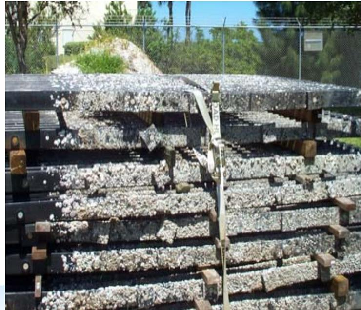
Fouling on intake trash gates **prior to installation** of FR coating system
